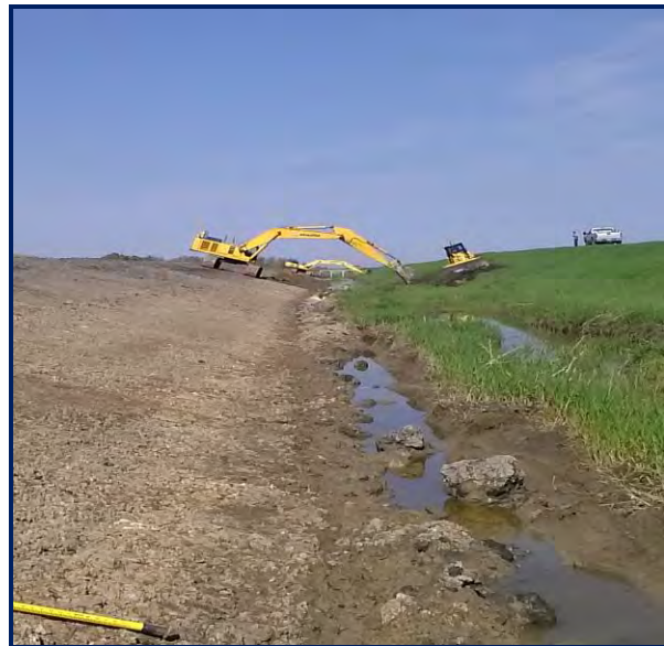
Channel excavation in the first mile of the project.
