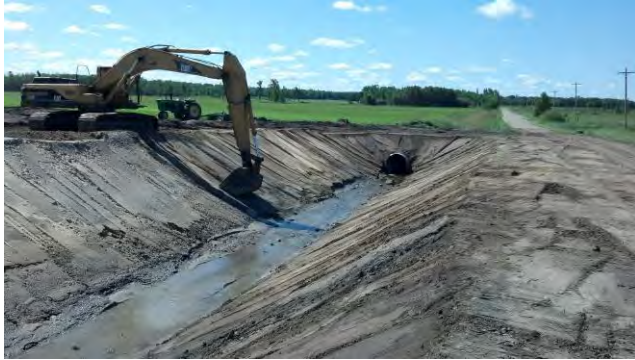
Looking South at repaired crossing and side slopes.
