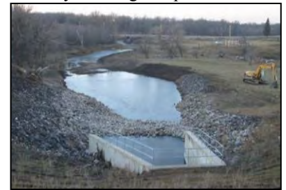
Looking downstream from outlet structure
