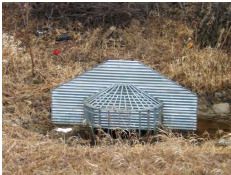
Cleaned trash rack.
