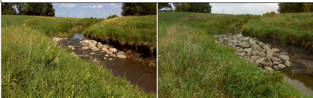
Photos of a rock check dam along AUID 515 immediately upstream of its confluence with the Grand Marais Creek on July 30, 2014 (left) and September 24, 2014 (right).
