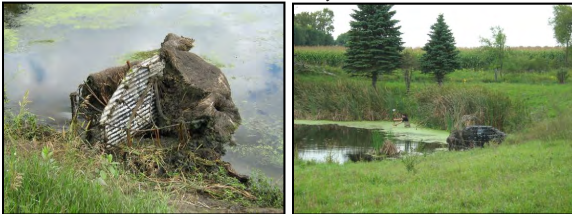
Miller Dam - Red Lake County – Pool Control Structure
