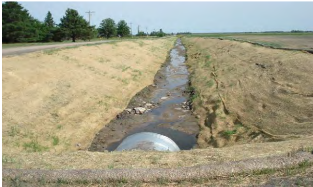
Looking south at repaired side slopes and mulch.
