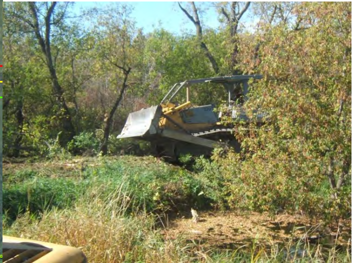
Contractor clearing trees in order to install side water inlets.
