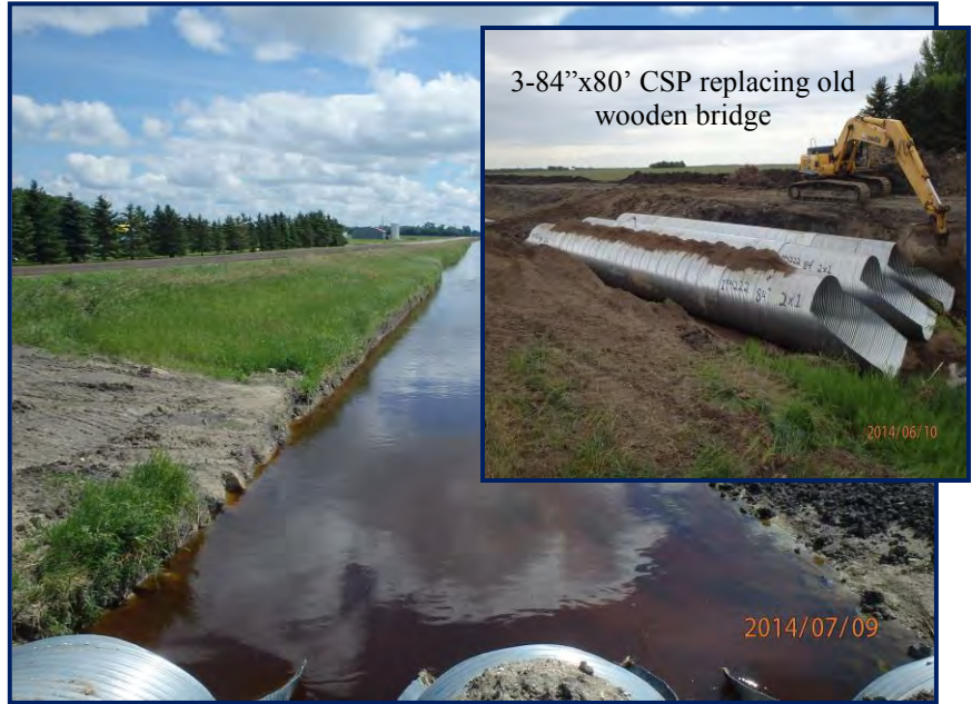
Finish work complete. Ready for seeding.
