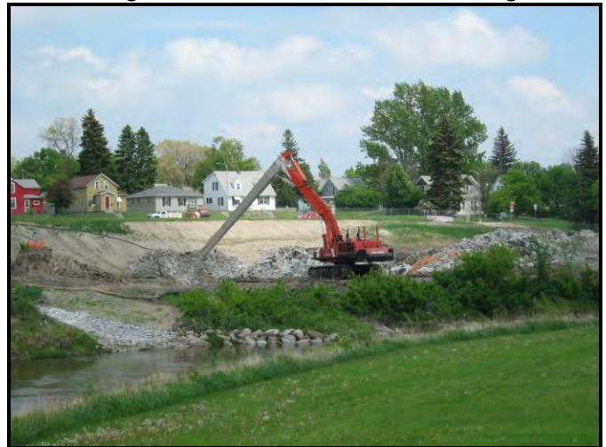
U.S. Highway #2 & Red Lake River at Crookston: MnDOT project – river bank slump was threatening the highway. Picture shows excavating one of 10 vertical walls on 'outside bank' – walls are 4' wide, 50' to 100' in length and an average of 70' below ground where the backhoe is working.
