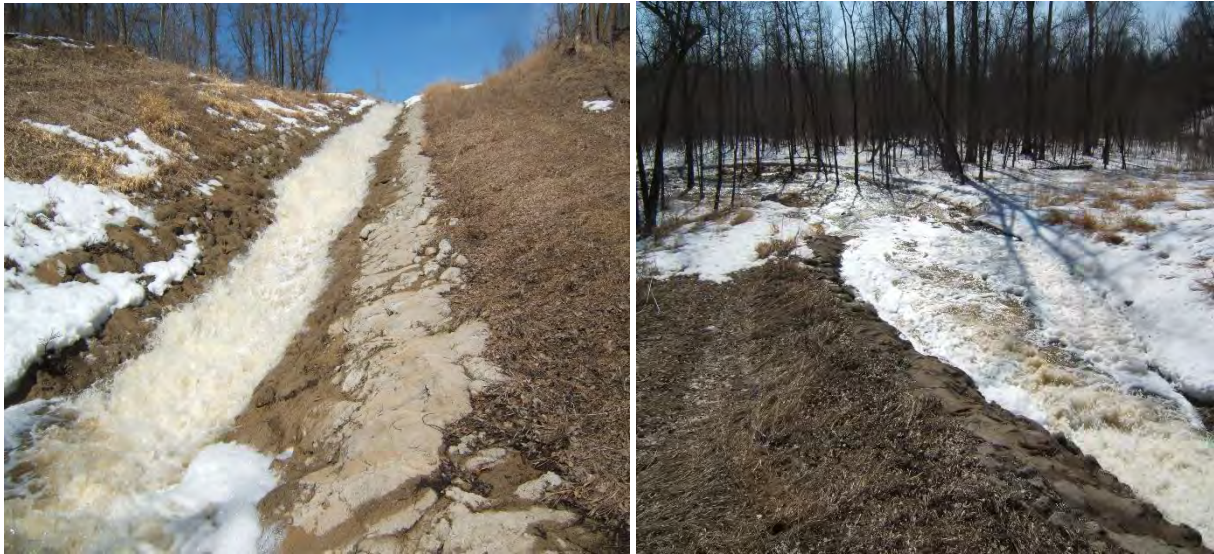
Spring runoff water flowing down the rock chute and into the plunge pool on RLWD Ditch 10.
