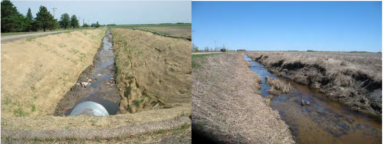
Repairs to Stabilize JD 72 Channel.
