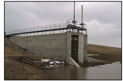
Principal outlet structure hydraulic gate operation
