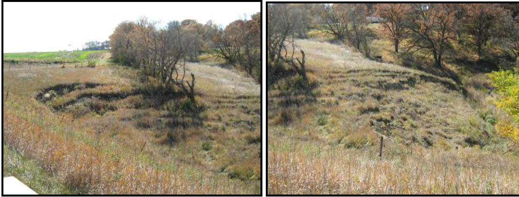
Latendresse Dam – Red Lake County – Slope failure & metal control structure has deteriorated
