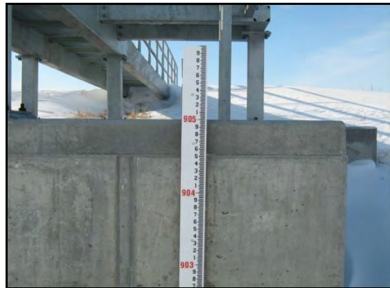
Typical staff gage at structure
