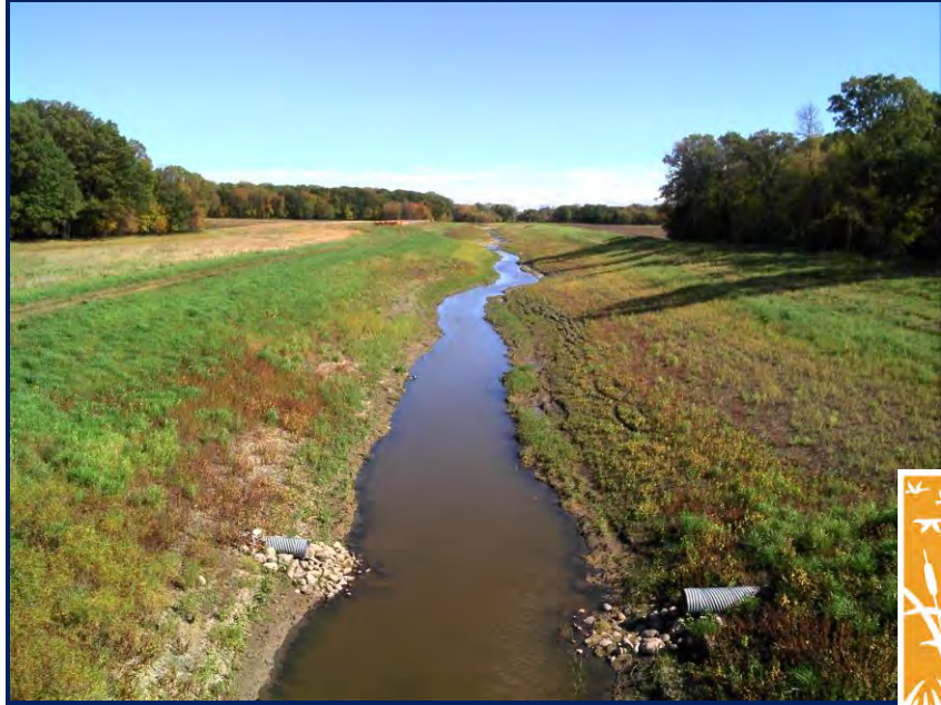
Stabilized channel looking upstream.
