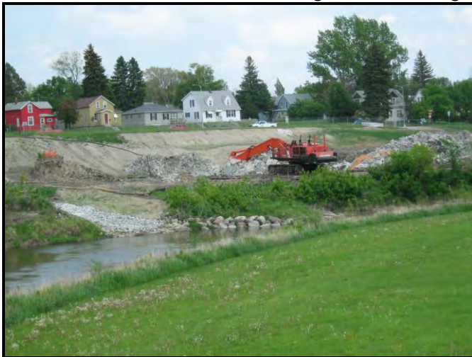
U.S. Highway #2 & Red Lake River at Crookston: MnDOT project – river bank slump was threatening the highway. Picture shows excavating one of 10 vertical walls on 'outside bank' – walls are 4' wide, 50' to 100' in length and an average of 70' below ground where the backhoe is working.
