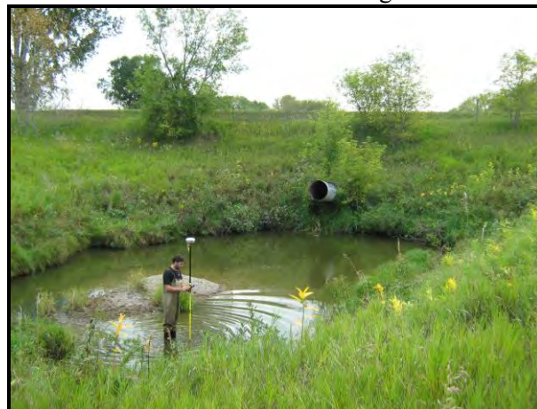
Miller Dam – Outlet / Plunge Pool
