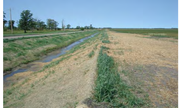
Looking north at seeded buffer strip.
