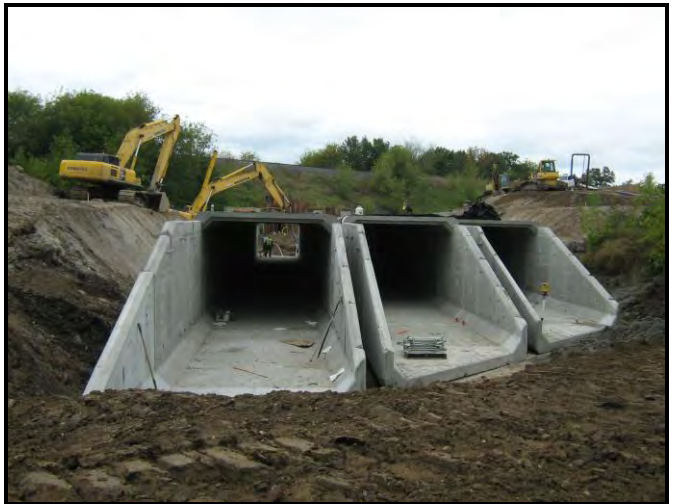
Lost River at U.S. Highway #59 near Brooks: MnDOT permit new culvert installation - 3 lines of 12' x 10' boxes.
