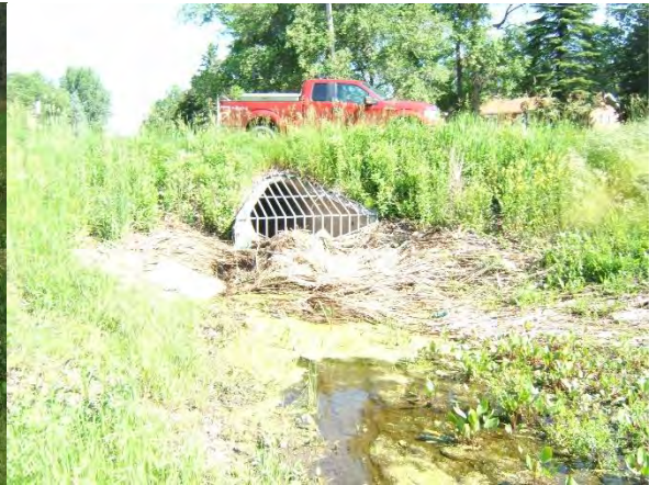
Trash that had to be removed at Greenwood Street.
