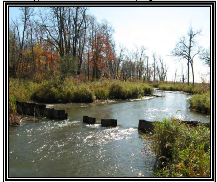
Typical Fall Drawdown with Stop-logs Removed
