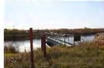
Figure 3 - Gated Outlet Structure - North Pool
