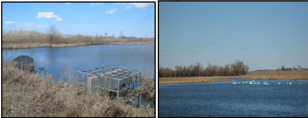
Odney / Flaot Dam - Polk County – scheduled for repair in 2016 – metal structure has deteriorated
