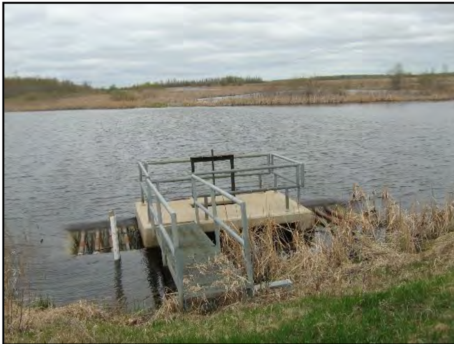
Pool Crest - June 18, 2015 – Elevation – 1173.5
