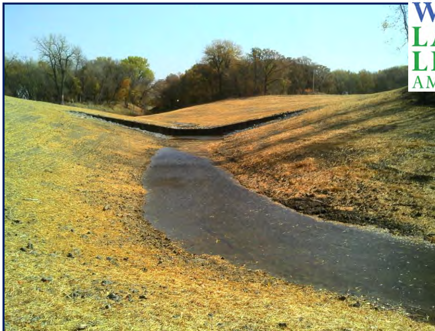
Drop structure looking downstream
