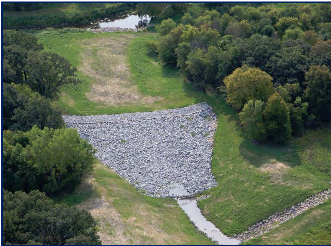
Cut Channel Outlet Structure – Phase II
