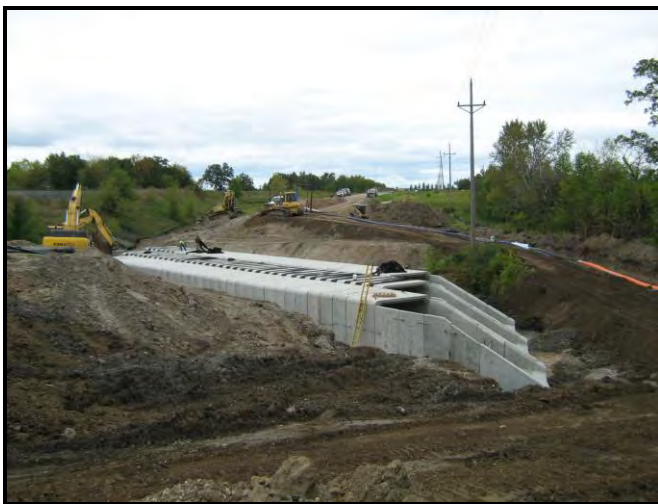
Lost River at U.S. Highway #59 near Brooks: MnDOT permit new culvert installation - 3 lines of 12' x 10' boxes.
