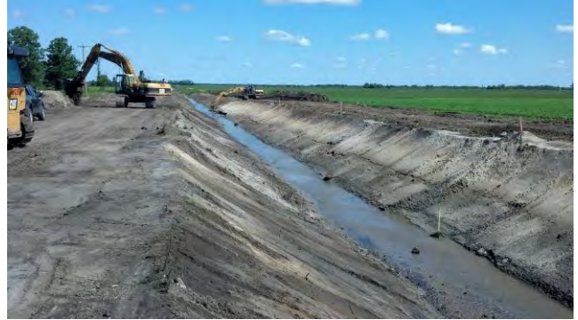
Looking north at repaired side slopes.
