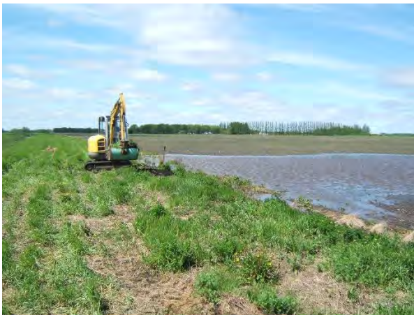
Cutting a hole in the berm to alleviate ponding water.
