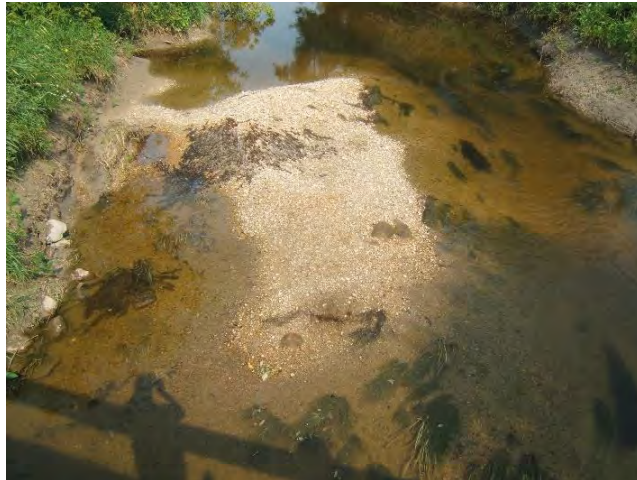
Silt bar in Channel.
