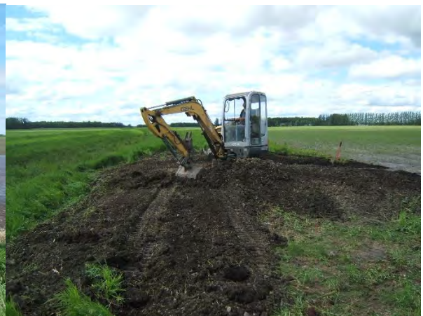
Final shaping taking place.
