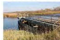
Figure 5 - Gated Outlet Structure - South Pool
