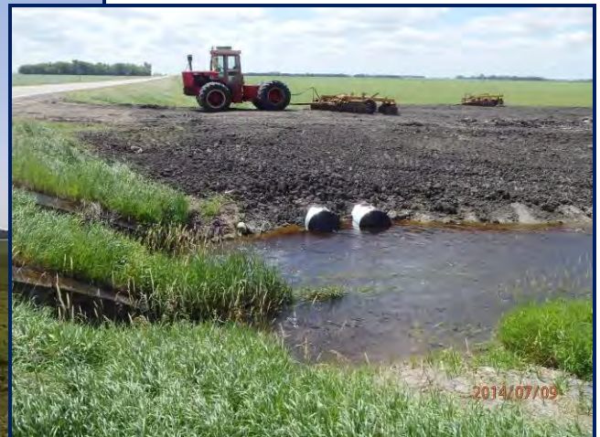
Side water inlet pipes installed. Finish work underway.
