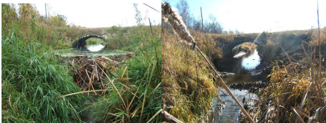
Dam located in Section 17, Greenwood Township along Clearwater County Road 5.
